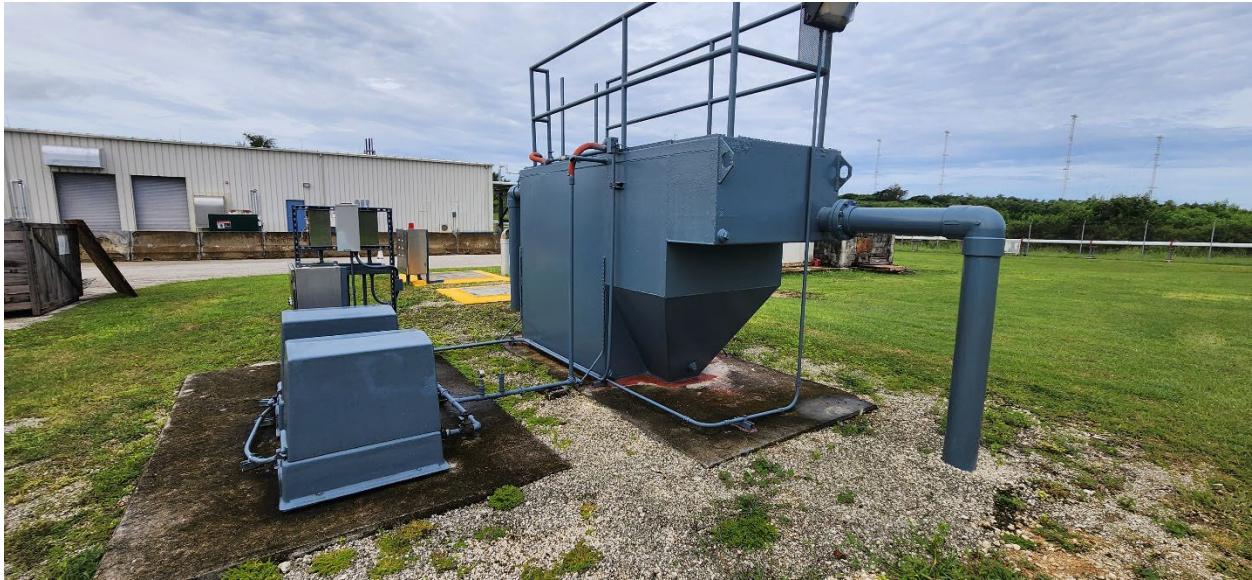
Figure 1. Existing Individual Wastewater Disposal System at USAGM
