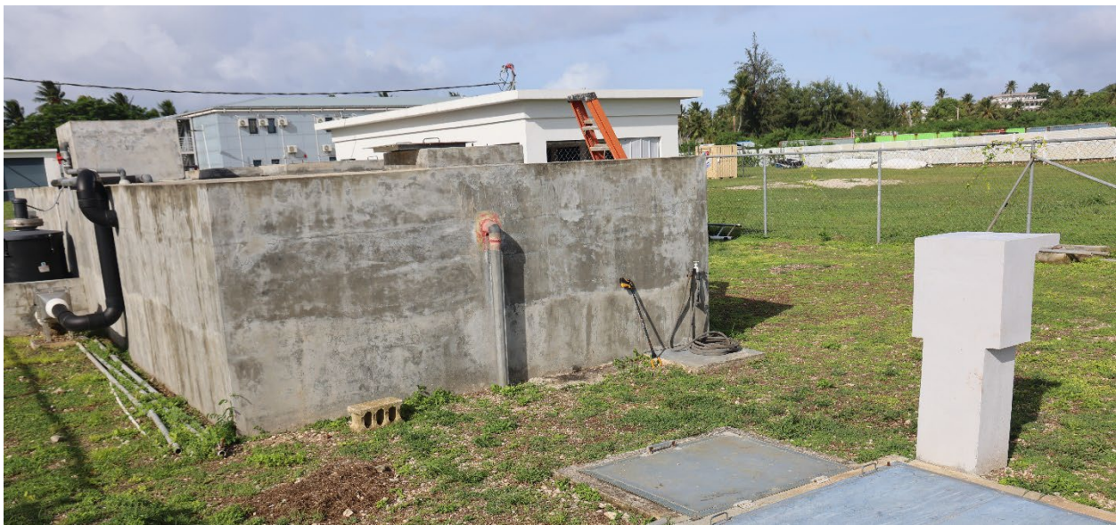
Figure 4 Other Wastewater Treatment System at Tinian Diamond Hotel and Casino
