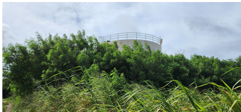
Figure 10 Marpo Tank (0.25 Million Gallons) in 2024
