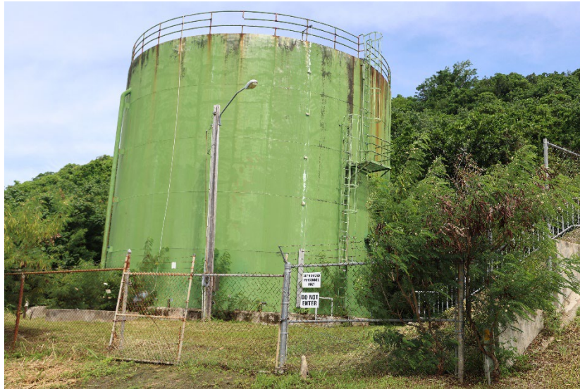
Figure 7 Carolinas Tank 1 (0.50 Million Gallons)
