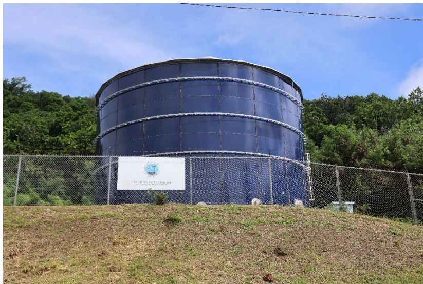
Figure 8 Carolinas Tank 2 (0.50 Million Gallons)
