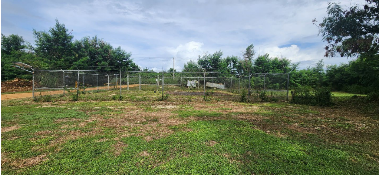
Figure 2 Existing Individual Wastewater Disposal System near Camp Tinian
