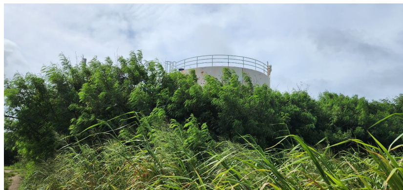
Figure 10 Marpo Tank (0.25 Million Gallons) in 2024
