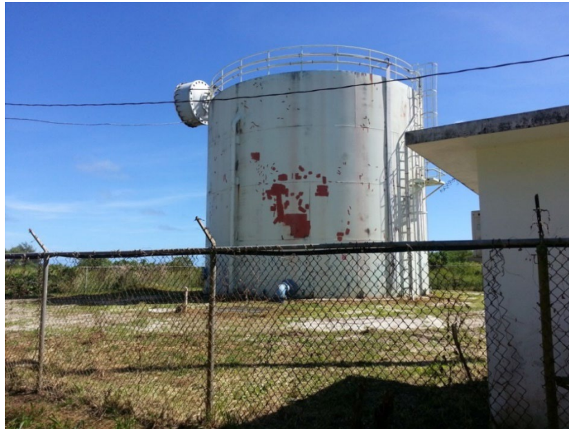
Figure 9 Marpo Tank (0.25 Million Gallons) in 2013
