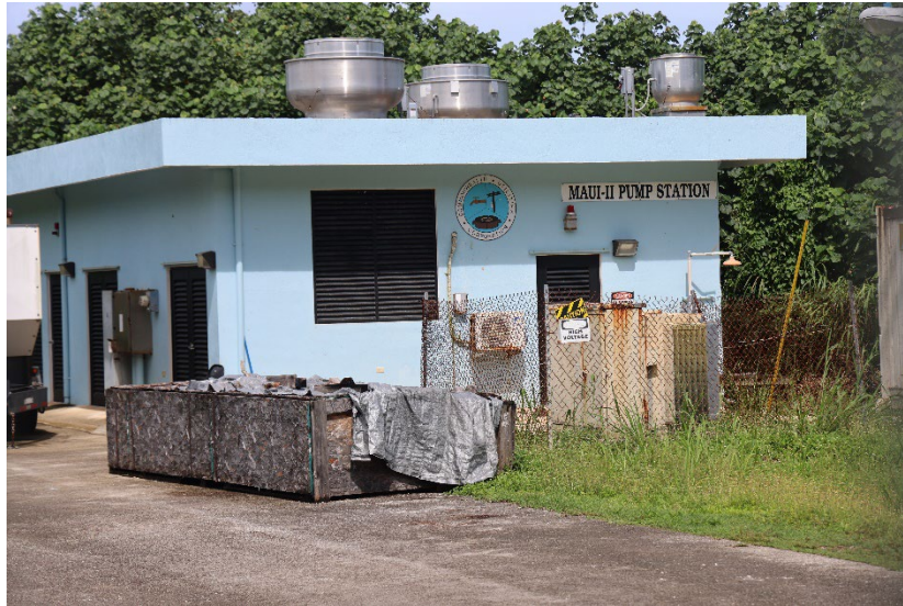
Figure 5 Maui Well No. 2 Pump House
