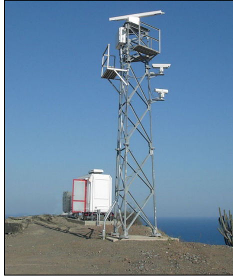
Figure C.4-1 Representative Surface Radar Tower
